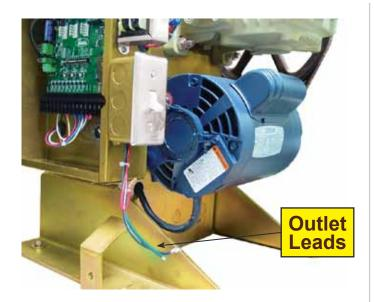
**Note:** 15 amp wires connected to independent breaker.
